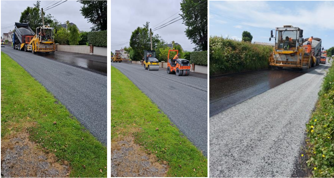
SURFACE DRESSING WORKS
