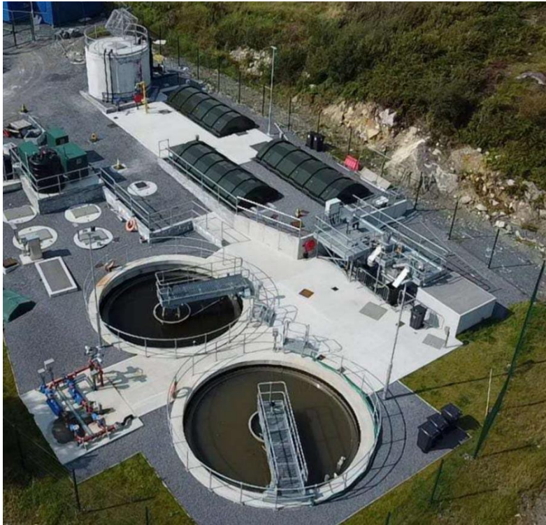
AN SPIDÉAL WASTEWATER TREATMENT PLANT
