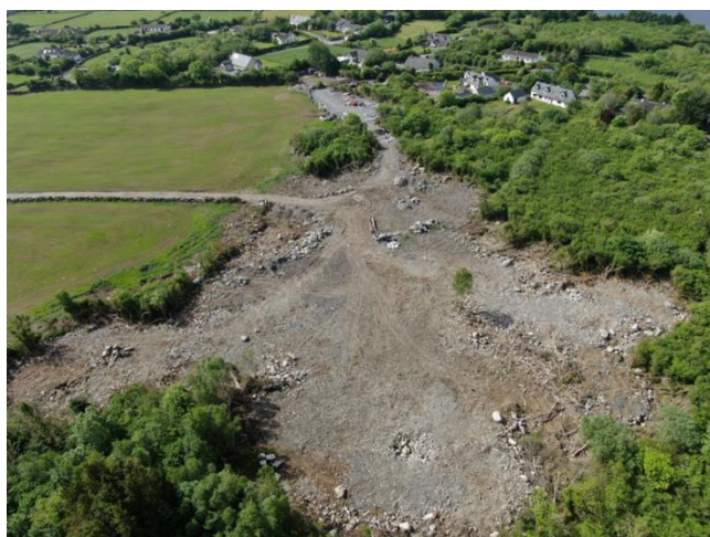
AERIAL PHOTO SHOWING THE SCALE OF UNAUTHORISED INFILL SITE.
