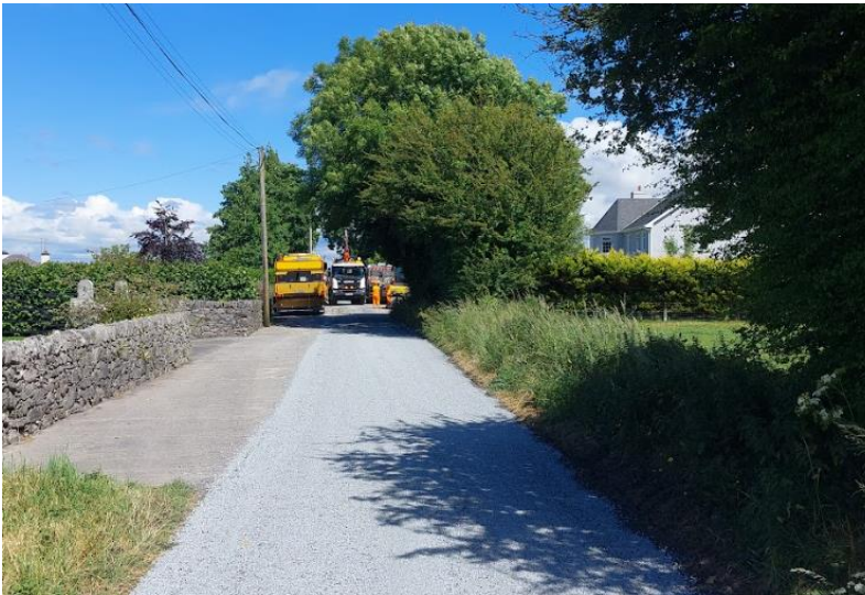
KILTROQUE, SURFACE DRESSING
