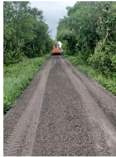
DURING ROAD RECYCLING WORKS TRI 16 L 6483 IRONPOOL
