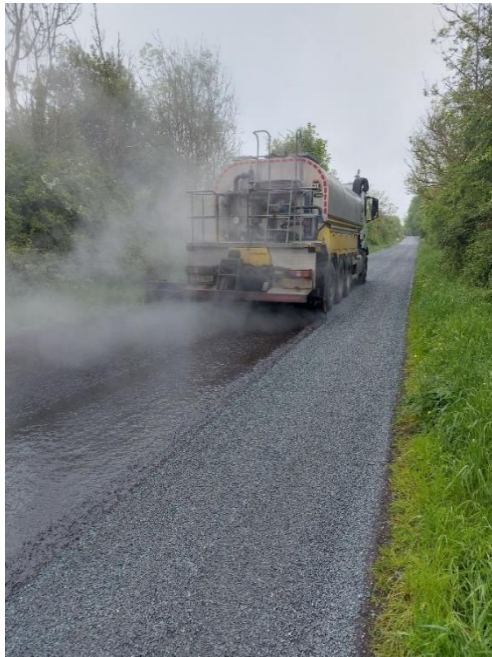
COLAS CONTRACTORS - RM SURFACE DRESSING, AT KILLUREMORE - 2024 ROADWORKS PROGRAMME BALLINASLOE MD
