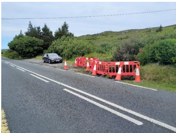
CONSTRUCTION WORKS FOR NEW GATEWAY SIGN ON N59 WESTPORT
