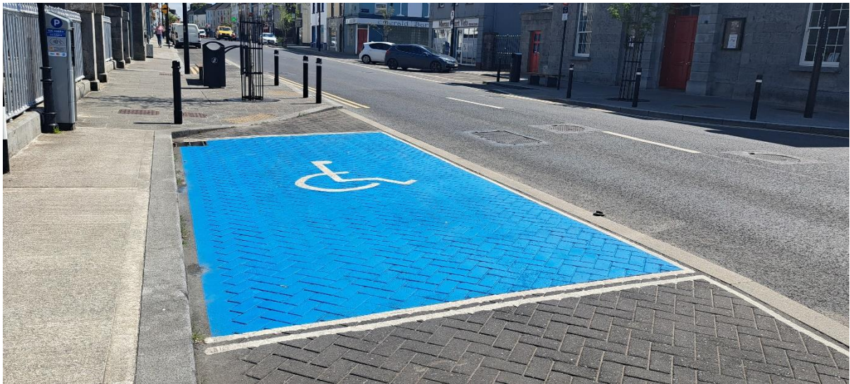
EXAMPLES ABOVE OF THE 7 NO. DISABLED PARKING BAYS ON MAIN STREET, DUNLO STREET & JUBILEE STREET, BALLINASLOE HAVE HAD UPGRADED MARKINGS APPLIED
