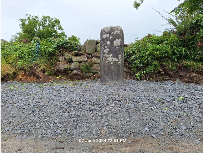
MILESTONE UPGRADE WORKS AT KILTARTAN
