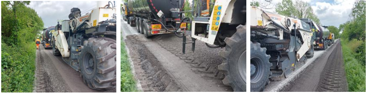
STABILISED ROAD RECYCLING AT DERREW, KILLIMOR
