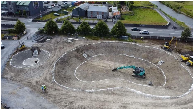
EXCAVATION OF ATTENUATION POND AT BAILE CHLÁIR
