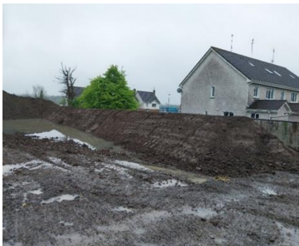
CONSTRUCTED BERM TO CONTAIN WASTEWATER
