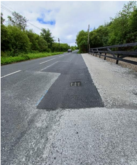
DRAINAGE WORKS RECENTLY COMPLETED ON LP-1320 AN SPIDÉAL/MAIGH CUILINN
