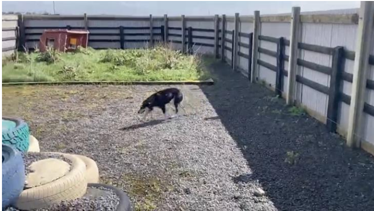
SHEETING INSTALLED IN OUTDOOR AREA
