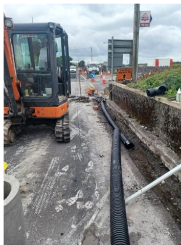
CLIMATE ADAPTION WORKS BALLYGADDY ROAD TUAM
