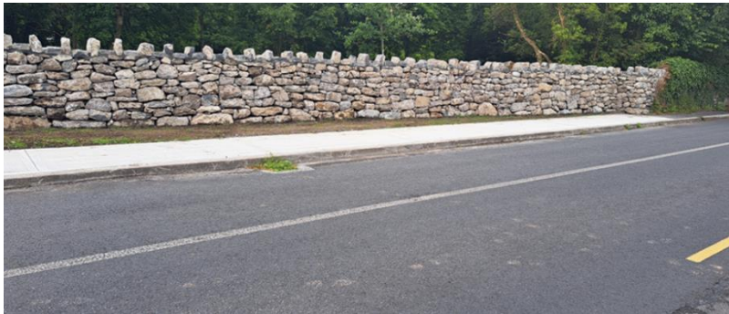
RENVILLE JUNCTION – ROAD SAFETY WORKS
