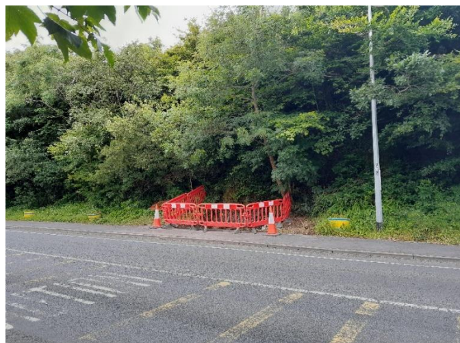
CONSTRUCTION WORKS FOR NEW GATEWAY SIGN ON R341 APPROACH
