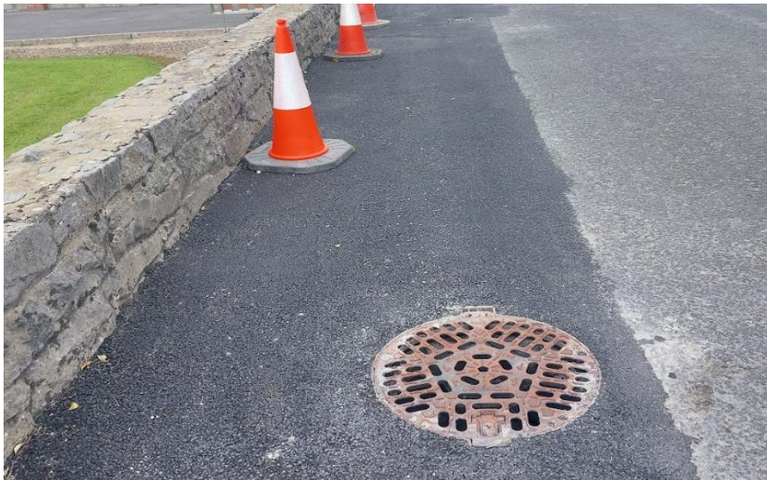
BALROBUCK DRAINAGE WORKS
