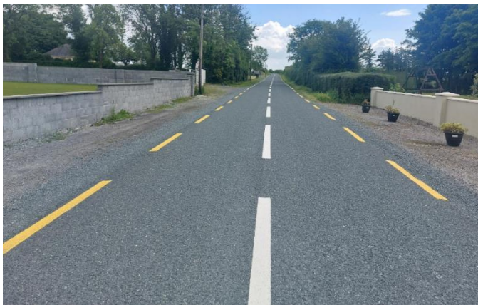
NEW ROAD LINING ON THE L4300, KILRICKLE TO MULLAGH ROAD FOLLOWING SURFACE DRESSING
