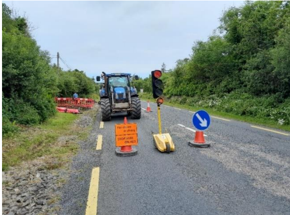
CONSTRUCTION WORKS FOR NEW GATEWAY SIGN ON N59 GALWAY APPROACH.
