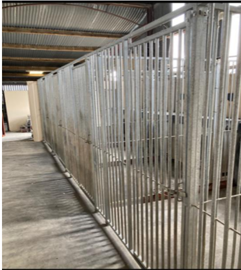
KENNELLING AREA PRIOR TO UPGRADE WORKS
