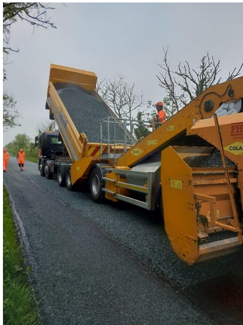
COLAS CONTRACTORS - RM SURFACE DRESSING, AT KILLUREMORE - 2024 ROADWORKS PROGRAMME BALLINASLOE MD
