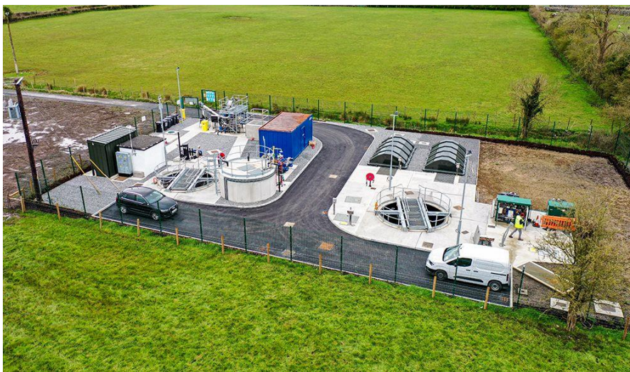
AHASCRAUGH WASTEWATER TREATMENT PLANT
