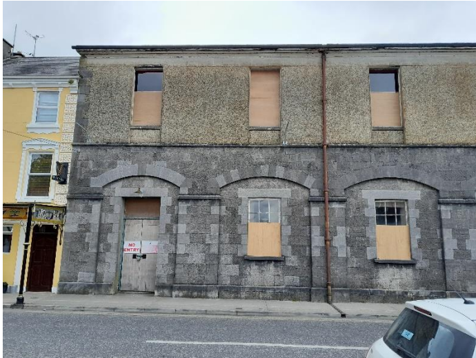
HOARDINGS TO WINDOWS WAS REPLACED FOLLOWING RECENT STORM DAMAGE.
