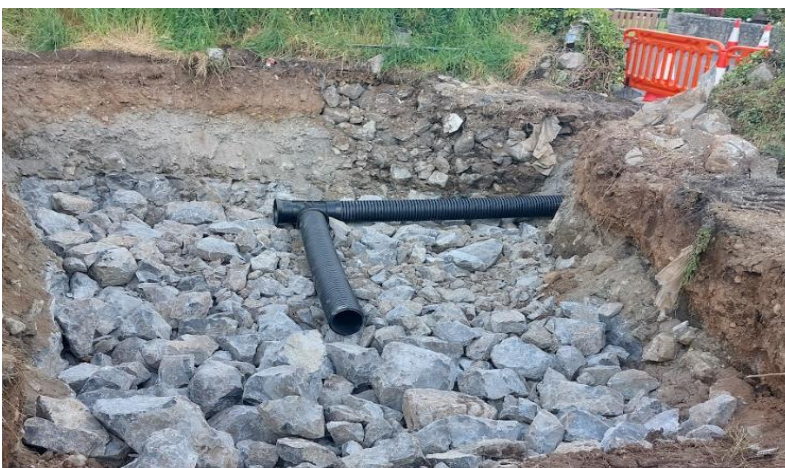
BALROBBUCK DRAINAGE WORKS
