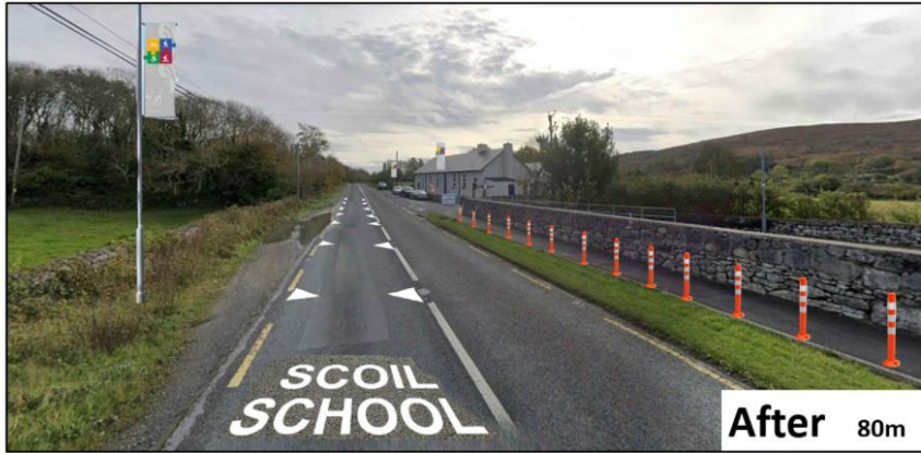
Fig. 5 – Artists Impression of ‘Sharks Teeth’ road marking and the ‘School/SRTS branding banner/totem.
